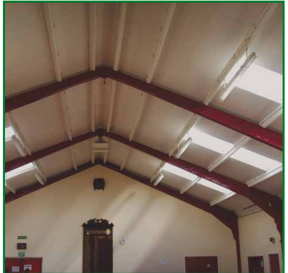
Penketh Pool benefitted from a £30,000 WREN grant to replace its roof
